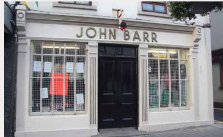
John Barr's drapery shop on Main Street, Bunclara exhibits many of the classic architectural features of a traditional shopfront Photograph: Joseph Gallagher
